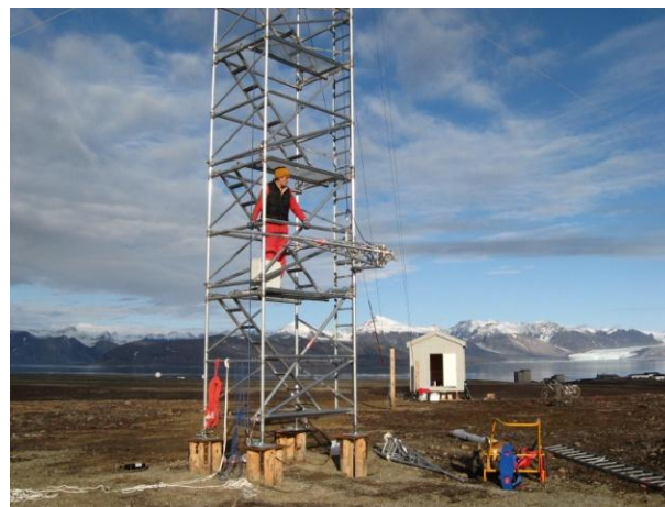
Photo 3: Beginning of installation – tests of rotating booms for radiometers
