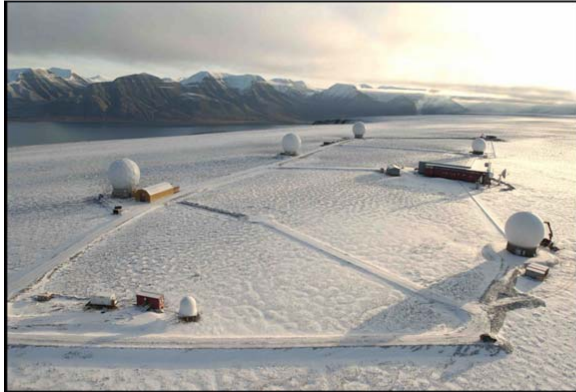
Sval Sat facilities
